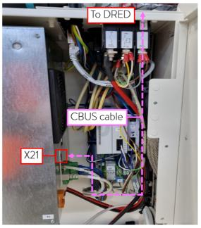
To achieve this, a data cable must be passed through from the DRED to X21 via the top plate of the sonnenBatterie Hybrid 9.53, preferably through a 20mm gland fitted to the blind grommeted hole labelled "S1" as per the image below.
